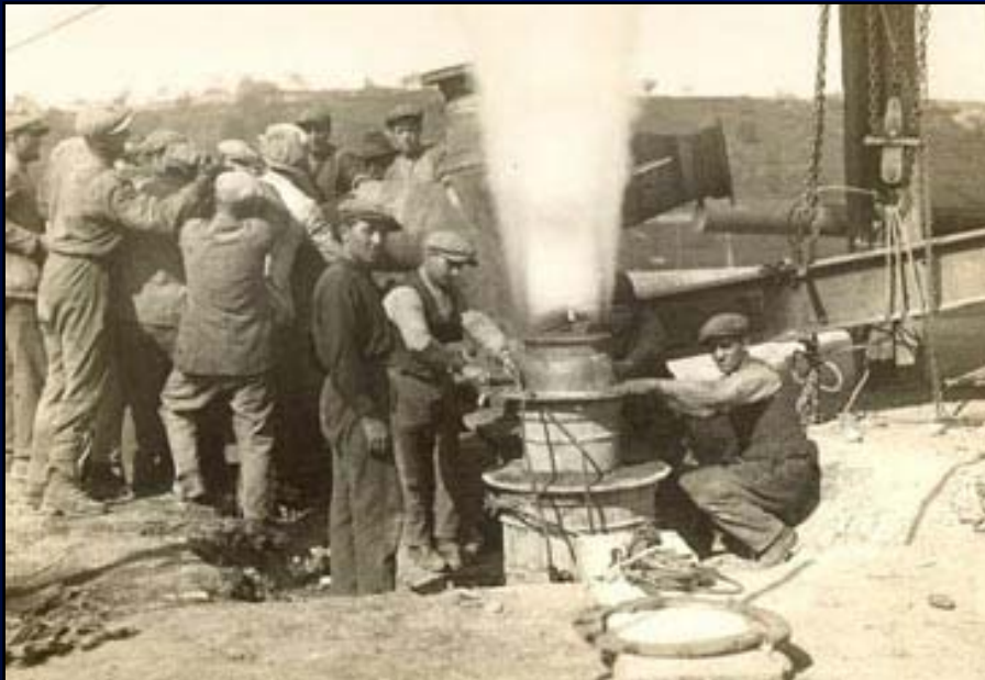
Photo: Tuscan Construction Crew, Larderello Geothermal Field
